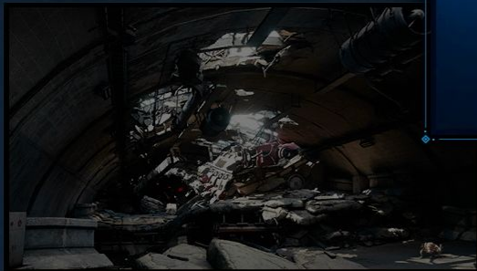
Collapsed Expressway - Entrance
